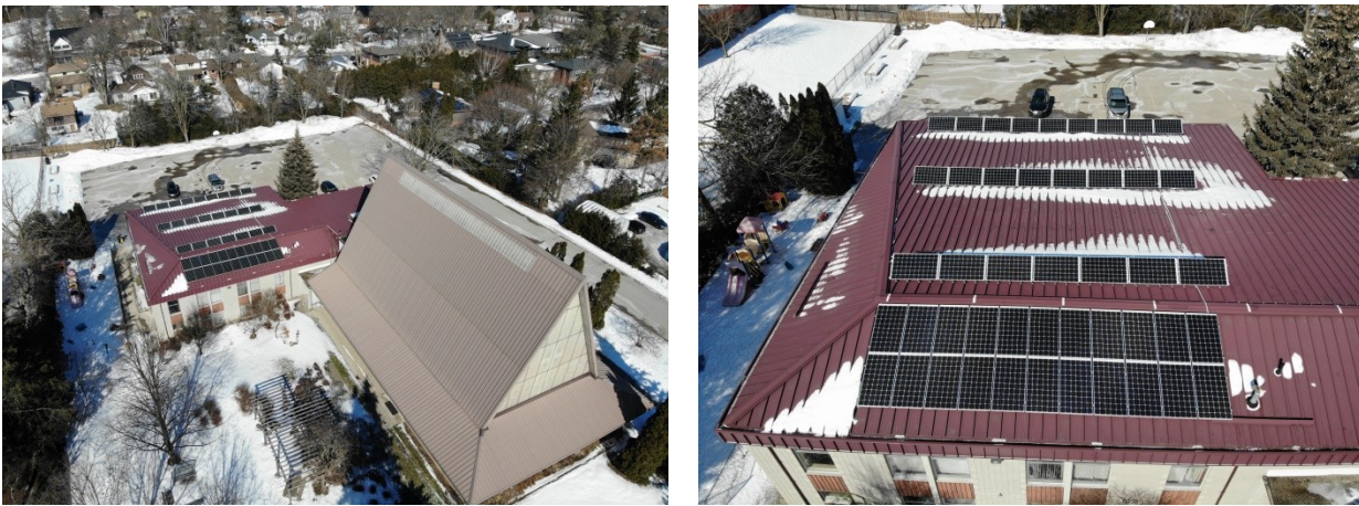
Above: Harcourt UC Solar Array on roof of gym, Feb. 24, 2022.
